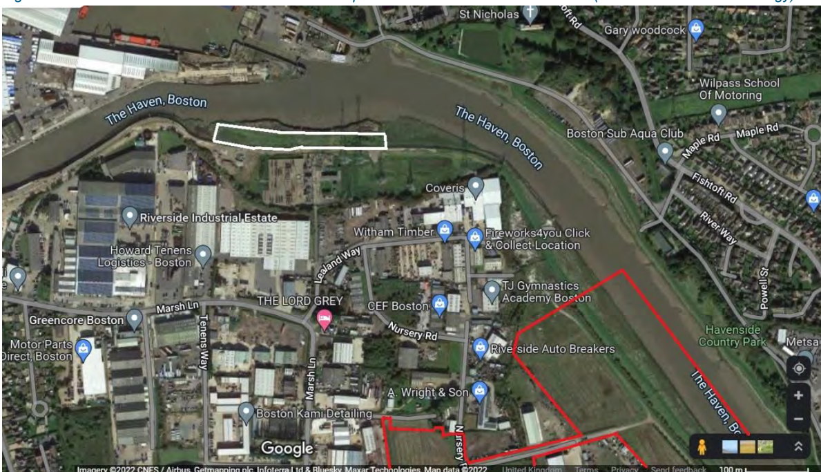
Figure 3 Annotated aerial view showing the indicative outline of raised land (within white polygon) behind sheet-pile wall in the bank, opposite Port of Boston lock on north side of The Haven. Principal Application Site lies within red line. (Imagery copyright 2022 Google, CNES / Airbus, Getmapping plc, Infoterra Ltd & Bluesky, Maxar Technologies, Map data copyright 2022)
