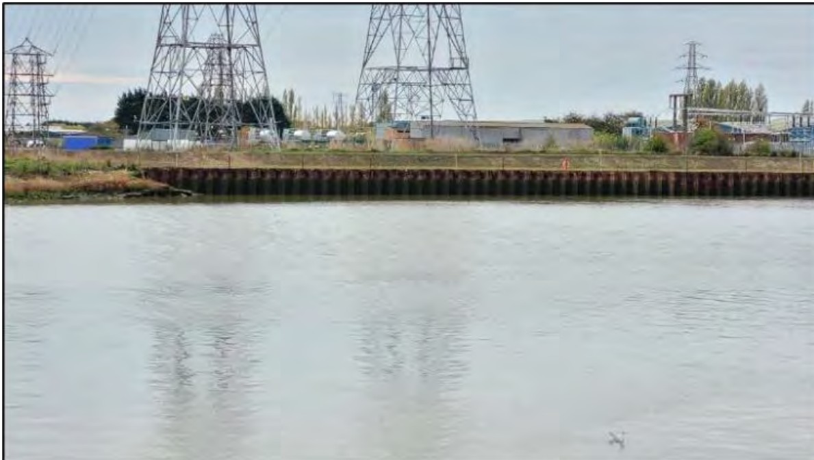
Figure 2 Ground view of securable land behind sheet-pile wall in south bank of The Haven (credit: Andrew Chick Ecology)
